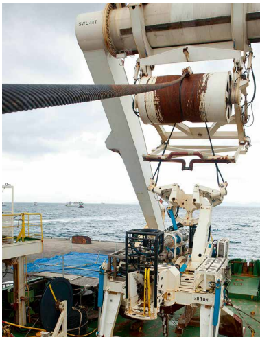
Laying submarine optical cable
