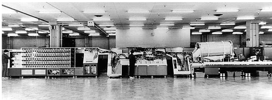
Automatic postal code reading-and-classifying machine
